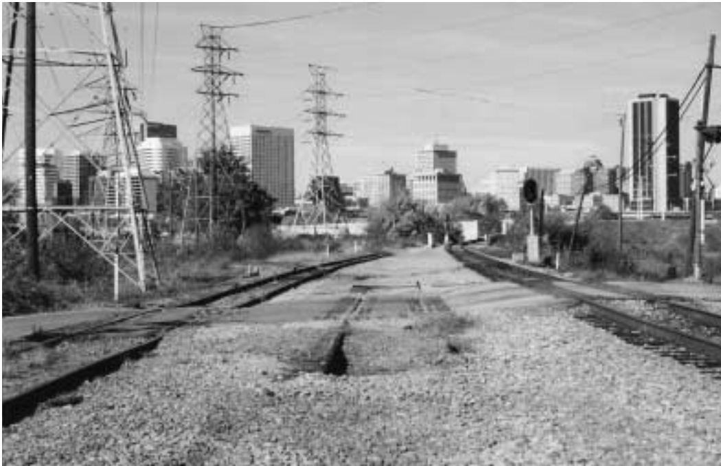
The CSX "S" Line approaching Richmond's Main Street Station. Note the previous track removal.
